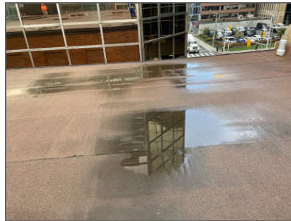
Figure 18 - Substation Roof Water Pooling
