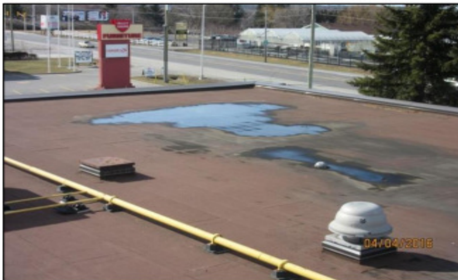
Figure 4 - 4565 Bank St (Water Pooling on Roof)
