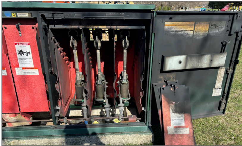
Figure 47 - UG Air Type Switchgear Failure
