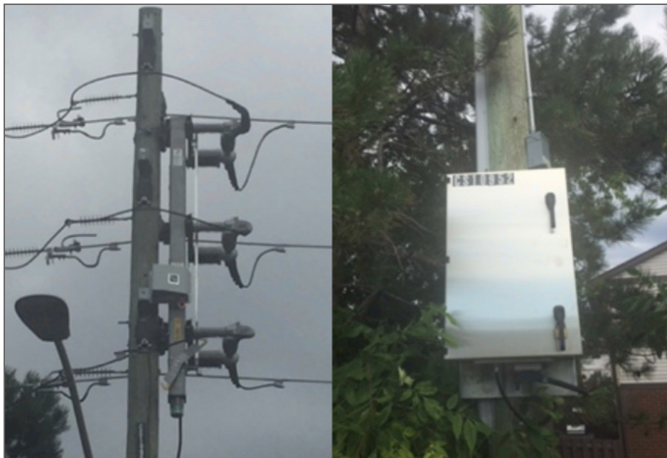
2 3 4 Figure 23 - Example of Smart FCI Device on Overhead Pole Line
