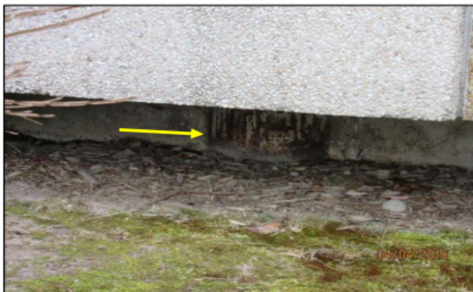
Figure 5 - 4565 Bank St (Spalling of Concrete Foundation )
