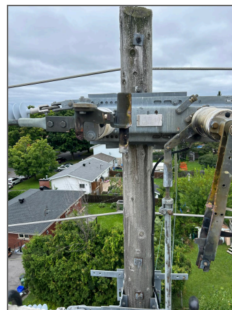
(b) Overhead switch operational defect
