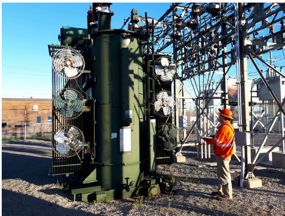
Figure 68 - Visual Inspection of a Station Transformer
