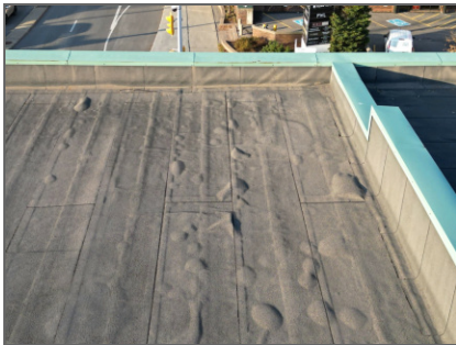
Figure 17 - Substation Roof Bubbling
