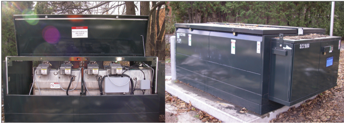
Figure 21 - Example of Automated Switchgear with Control Box
