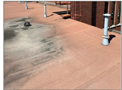
Figure 19 - Substation Roof Damage Caused by Water Pooling
