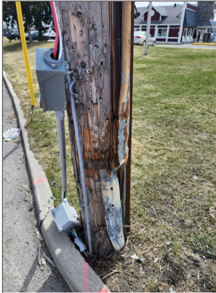
Figure 77 - Pole Damaged Due to Motor Vehicle Accident
