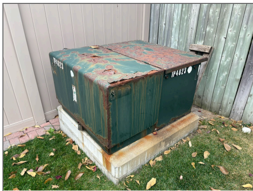
(a) Underground transformer corrosion
